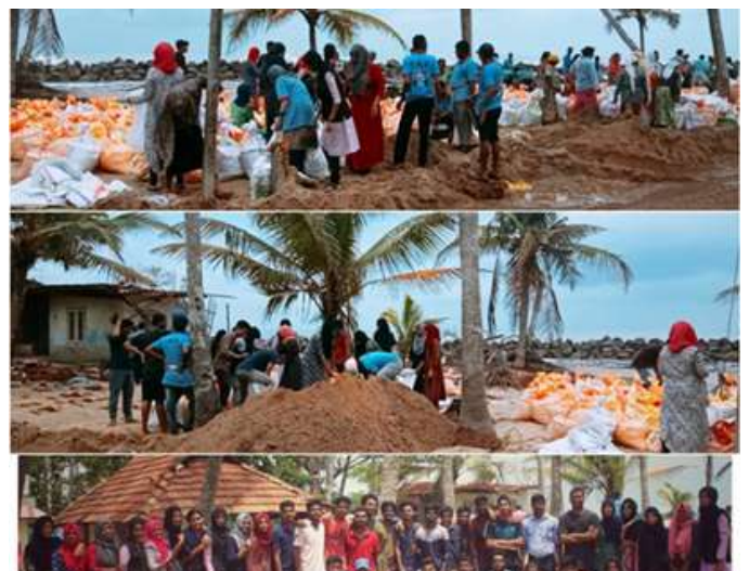
Sea wall making with sacks of sands
