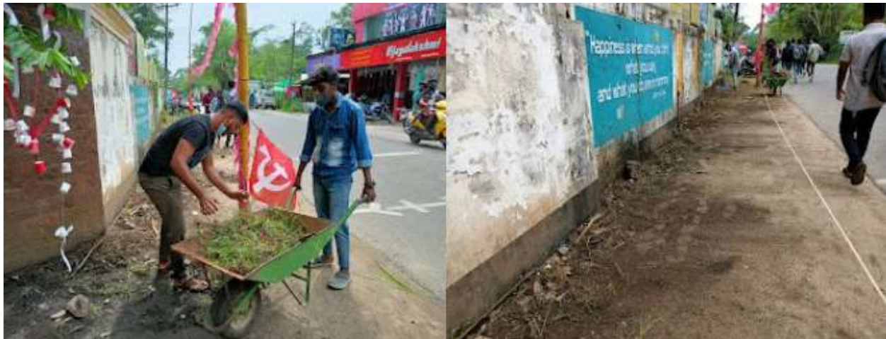
Campus Road Cleaning Work
