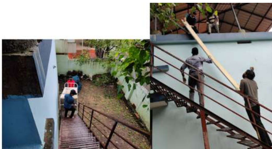
Primary Health Centre Cleaning Work 14 Nov 2021
