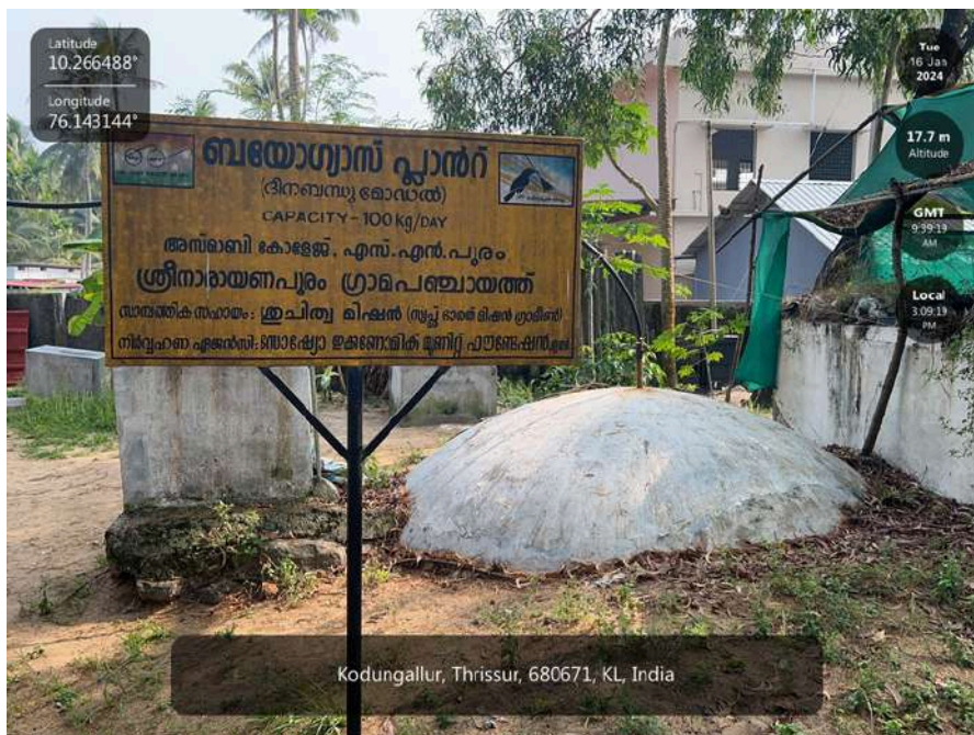
Biogas Plant in the College Hostel
