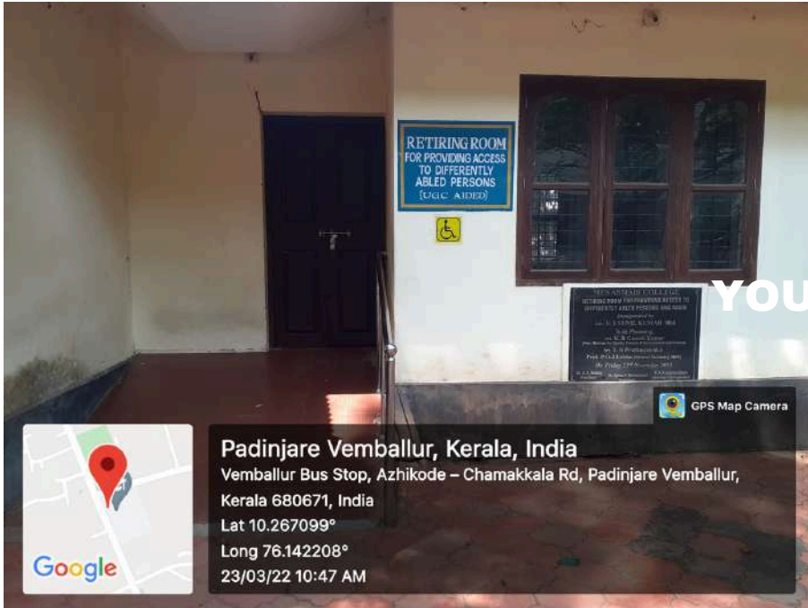
Retiring room for Differently Abled adjacent to the Main Building
