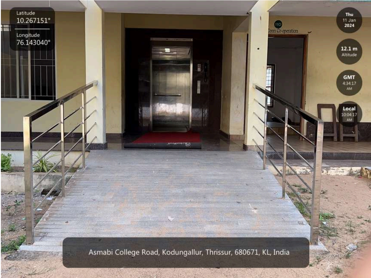
Ramp facility in the commerce block
