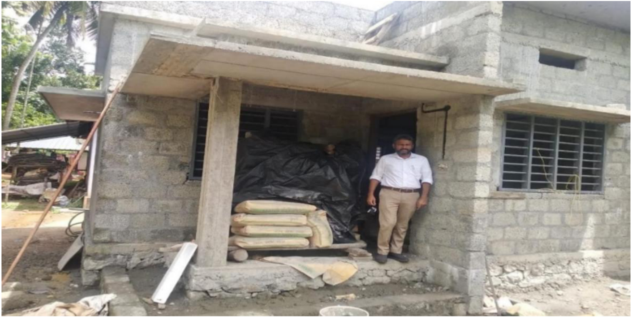
Construction of House for a student (Site Visit)
