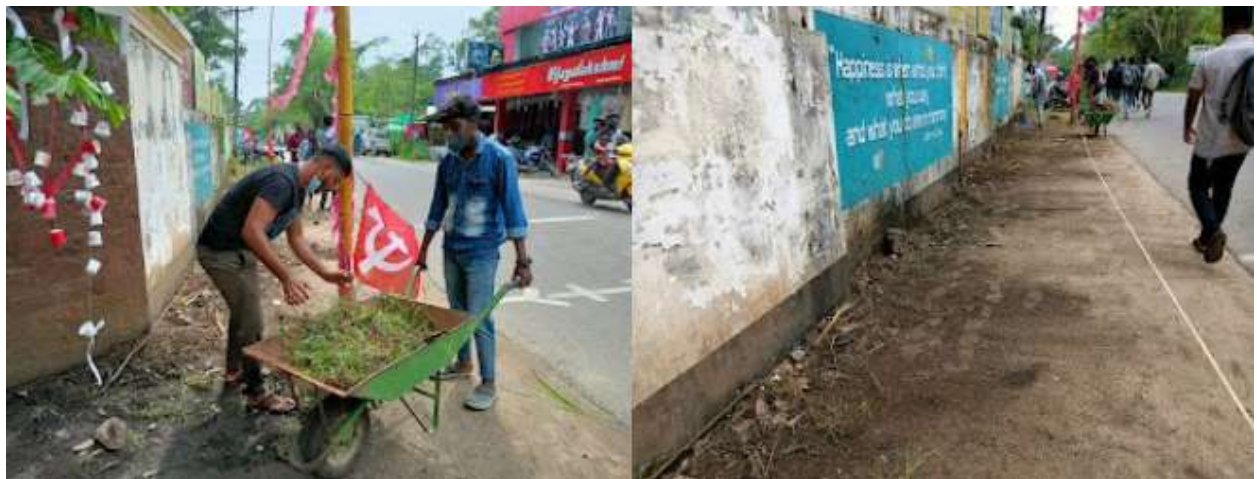
Campus Road Cleaning Work
