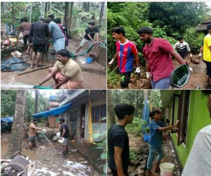
Flood Relief Activities
