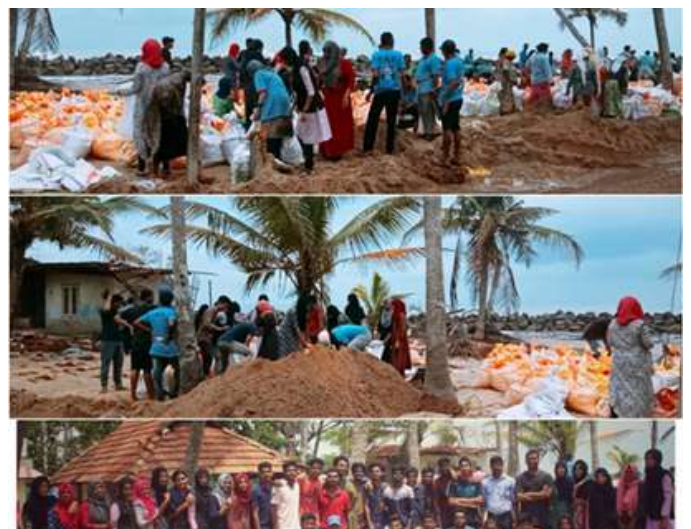
Sea wall making with sacks of sands
